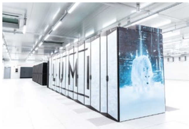
Figure 9.1. The beginning of building the LUMI High-Performance Computer in the new data center
