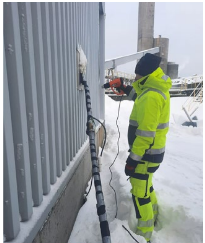
Figure 6.3. Piloting in winter conditions.
