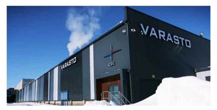
Figure 9.1. The CSC data centre in Kajaani is a global leader in energy conservation and cost-effectiveness, using 100 per cent hydropower with minimal cooling energy required due to the climate in Kajaani.
